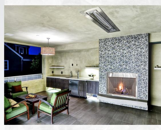
Bel Marmo Finish is a unique blend of marble dust, marble aggregate, and slaked aged lime, designed to achieve a classic Marmorino matte finish with either a smooth or distress texture. Inherently water-resistant and durable, Bel Marmo can be used on a variety of exterior and interior surfaces to create a unique and long lasting finish.
